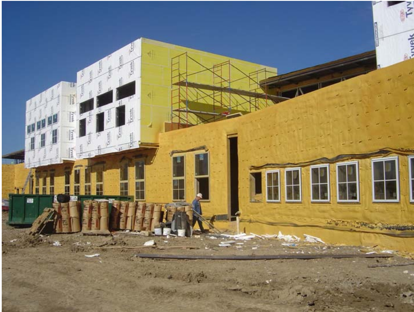
3" Sprayed-On Polyurethane Insulation
